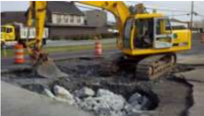
Photo 5 Shows a current (Spring 2011) on East Main St. (Rt. 422) in Palmyra
