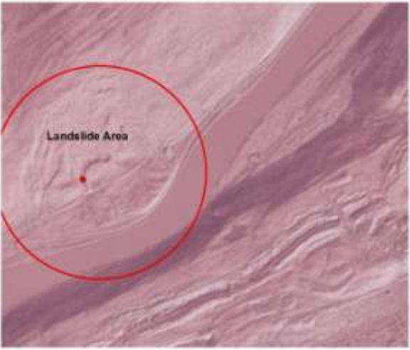
Figure 22 PAMAP aerial view of landslide area
